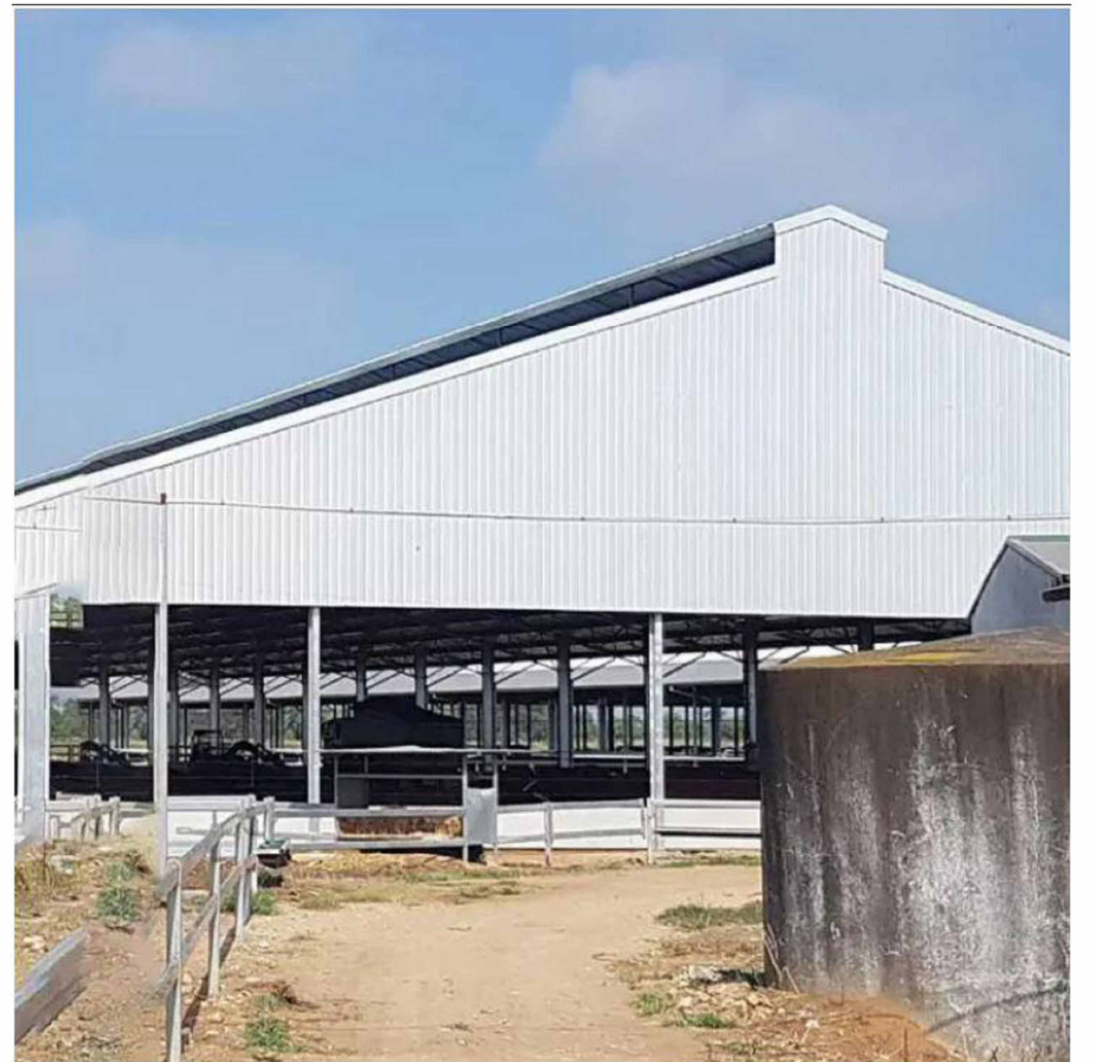
FIGURE 1. INDICATIVE ROOF WITH OPEN VENTILATION
