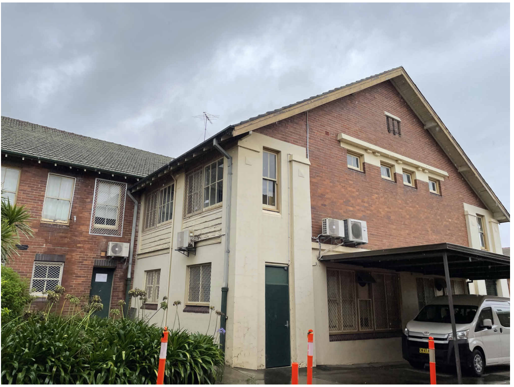
The south eastern corner of Building A viewed from Building B
