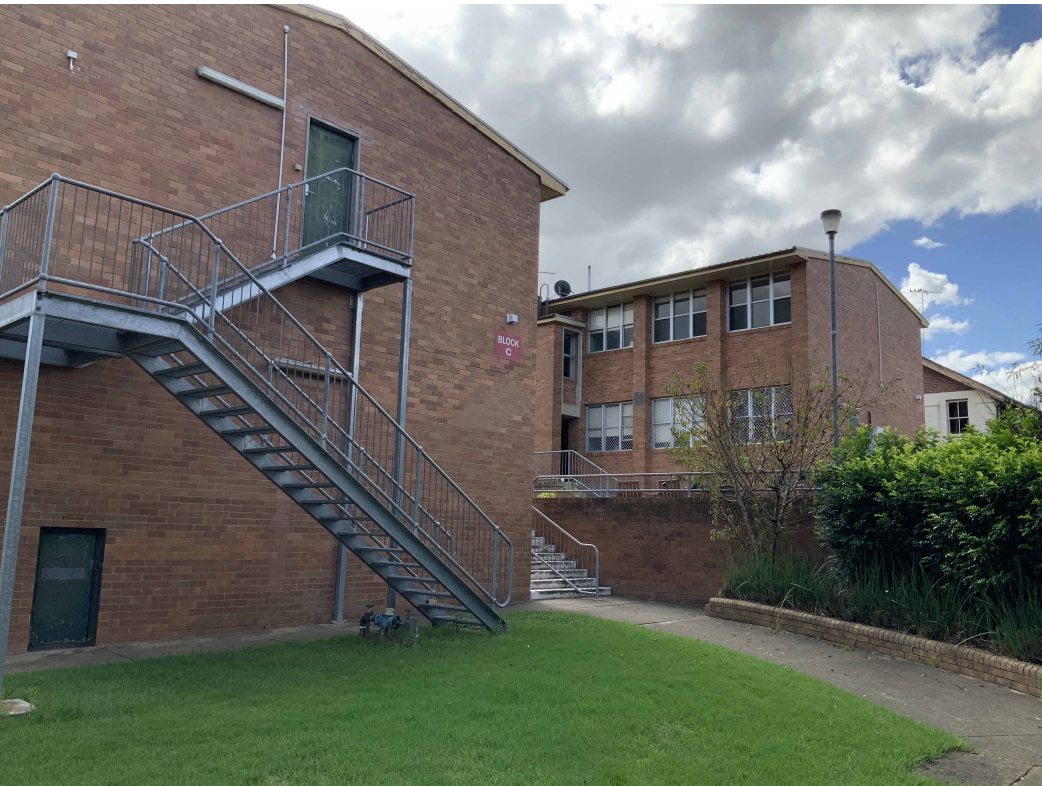
View of the existing Buildings B and C from the pathway leading out of the Wellness Centre (Building O)
