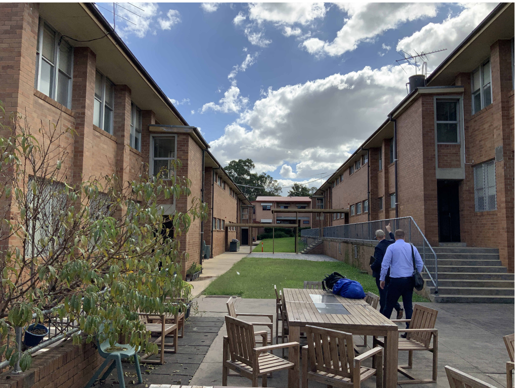
View of circulation space between Building B and C as seen from the open seating area in front of the Dining Hall (Building D)
