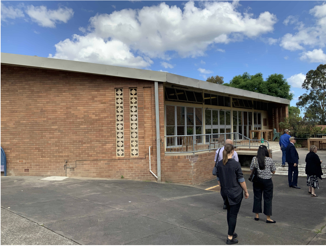
View of the entrance to the existing Dining Hall (Building D)
