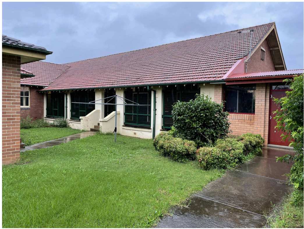
Photo of the existing verandah and connection to Building N
