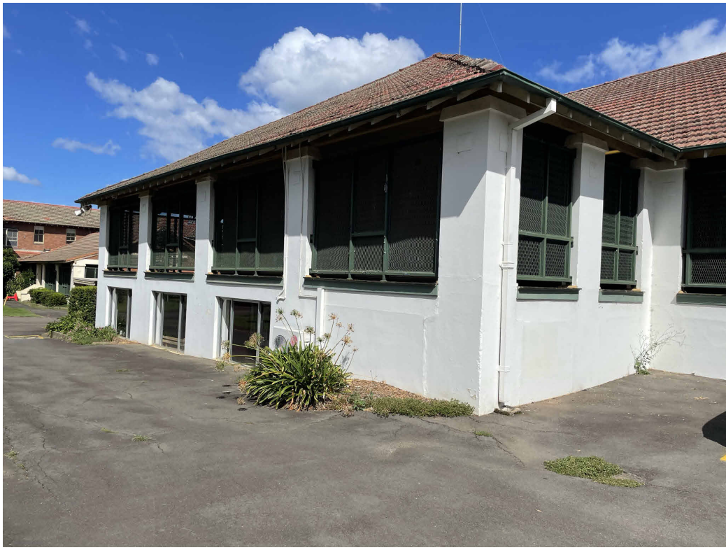
Photo of the verandahs on the northern facade of Building A
